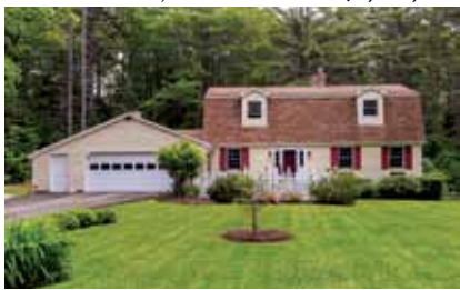
BOOTHBAY HARBOR WATER ACCESS
